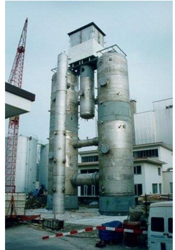
The Panda test facility built and operated by PSI in Switzerland.
